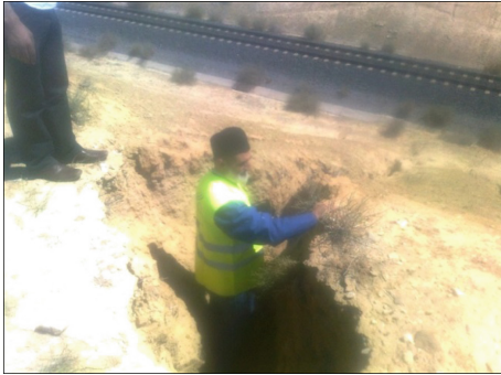
Fig. 2. Gullying in the slope crest
